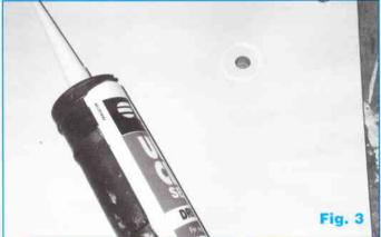
Use a caulking gun if you have one, to squeeze out a bead of silicon around each hole (**Fig. 3**) then lay each mesh square in place on the bead.
