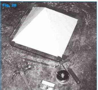
Pin the top ends of the roof panels together with 25 mm nails driven into adjoining roof panels.
